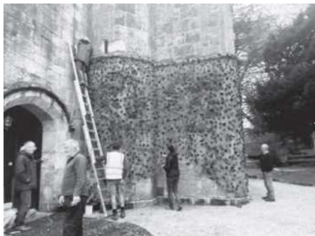
Preparing the Church Tower!
